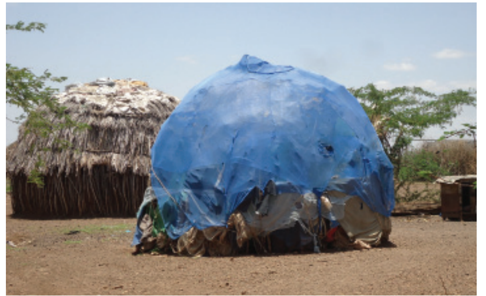
Manyatta house constructed with polythene paper in Kakuma Turkana west
